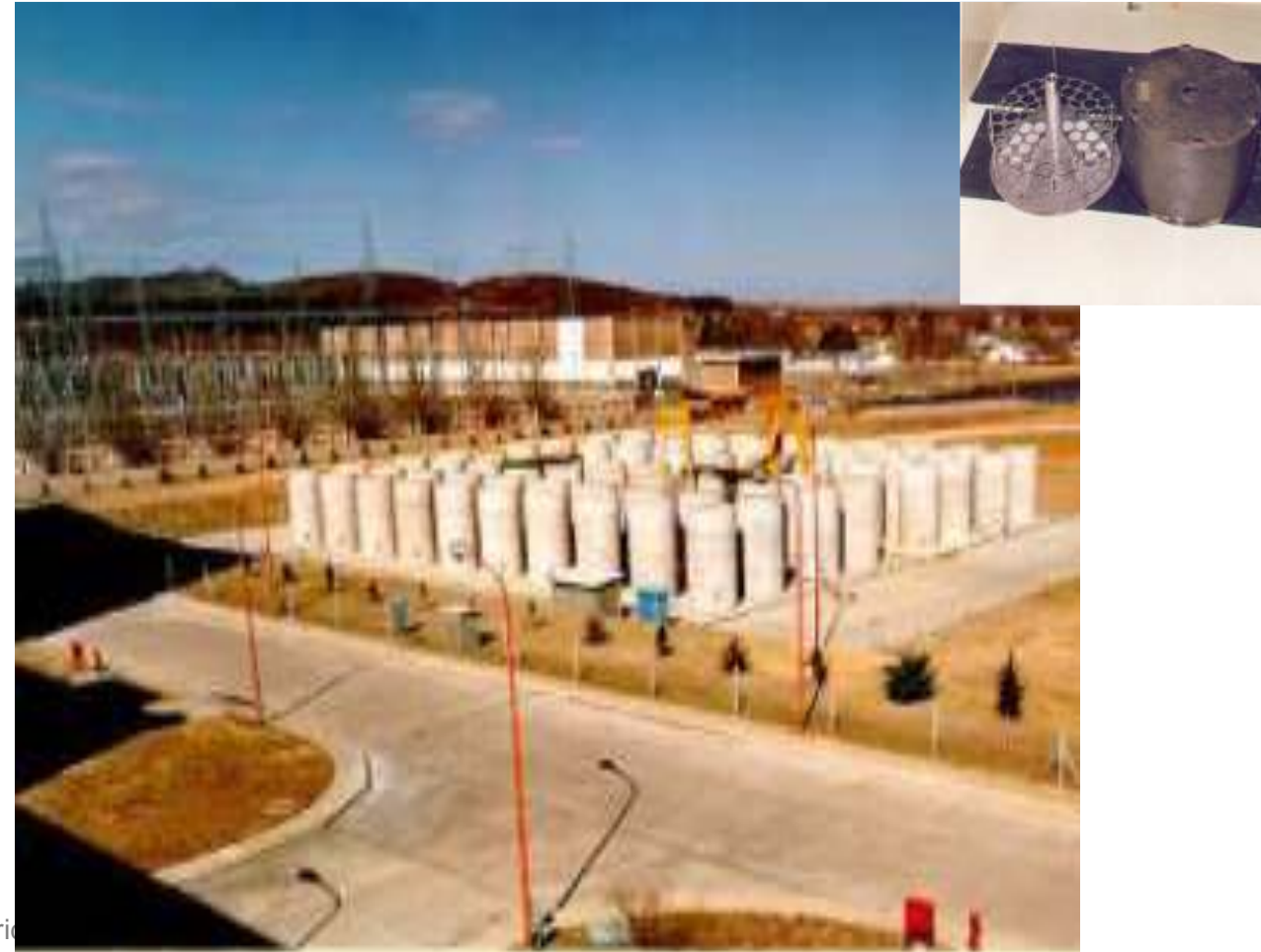
Embalse Nuclear Power Plant (CNE): Storage Silos (ASECQ)
