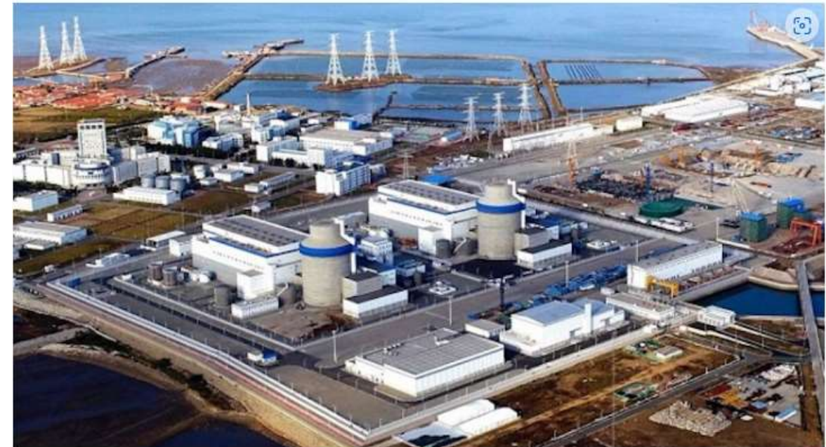
The Haiyang nuclear power station in China has two Westinghouse AP1000 plants.
