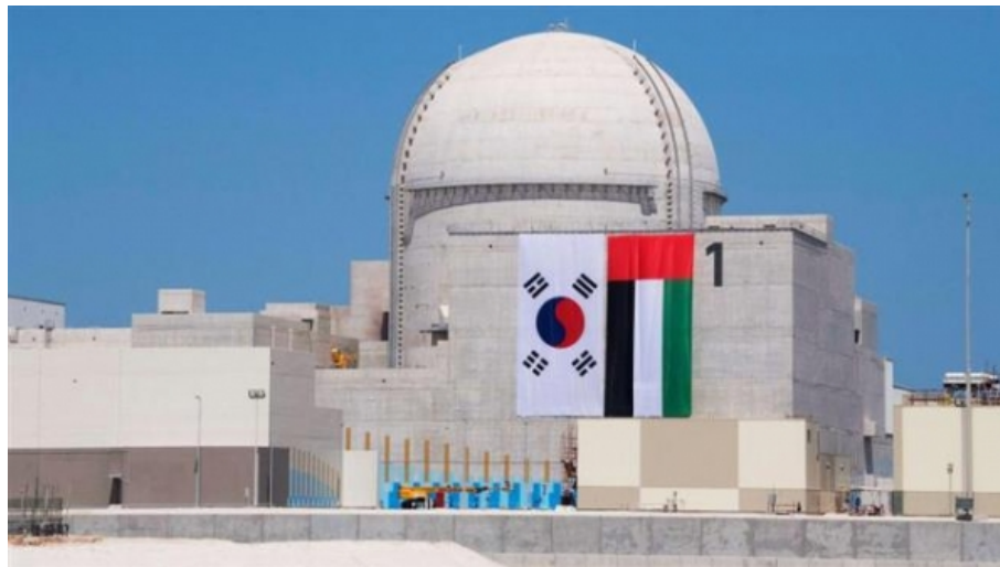
Barakah nuclear power plant
