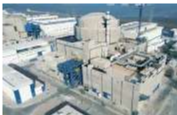
Fuqing 5 - China Hualong One In operation
