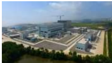
HTR-PM, China 2x110 MWe HTGR Under Commissioning
