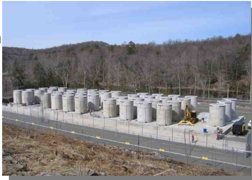
Dry cask storage for used fuel at the Surry station in Virginia
