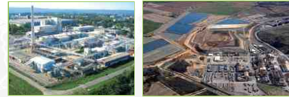
France: Comurhex Malvesi & Pierrelatte conversion facilities
