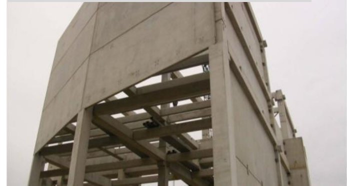
Cooling Tower 2A Structure – December 2012
