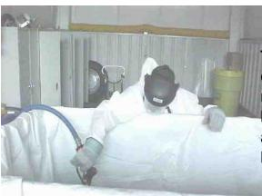
The waste is pure liquid and contains contaminants of radioisotopes. About 100 lbs of *Waste Lock® is* first added to the bottom of the box.
