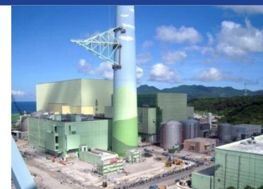
Under Construction COD 2013 (estimated)
