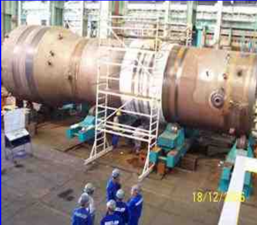
Local stress relieving heat treatment (electromagnetic induction)
