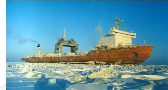
KLT-40 Icebreaker Reactor (35 MWe floating nuclear power plant)
