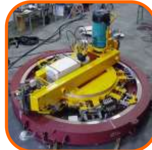
Machining of RPV flange
