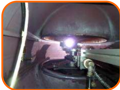
In-situ Valve Repair
