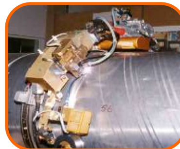
Welding of Aluminum pipes
