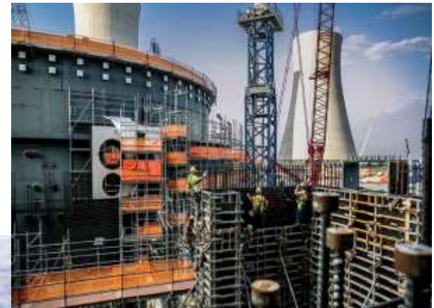
Vogtle Unit 3 Courtesy of Georgia Power
