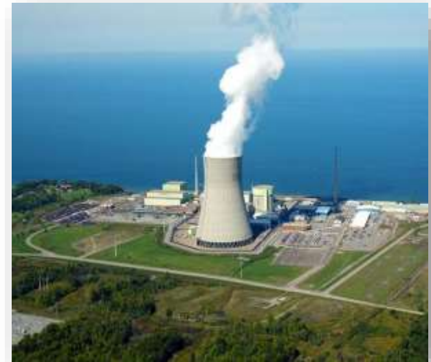
Nine Mile Point ~ Courtesy Exelon
